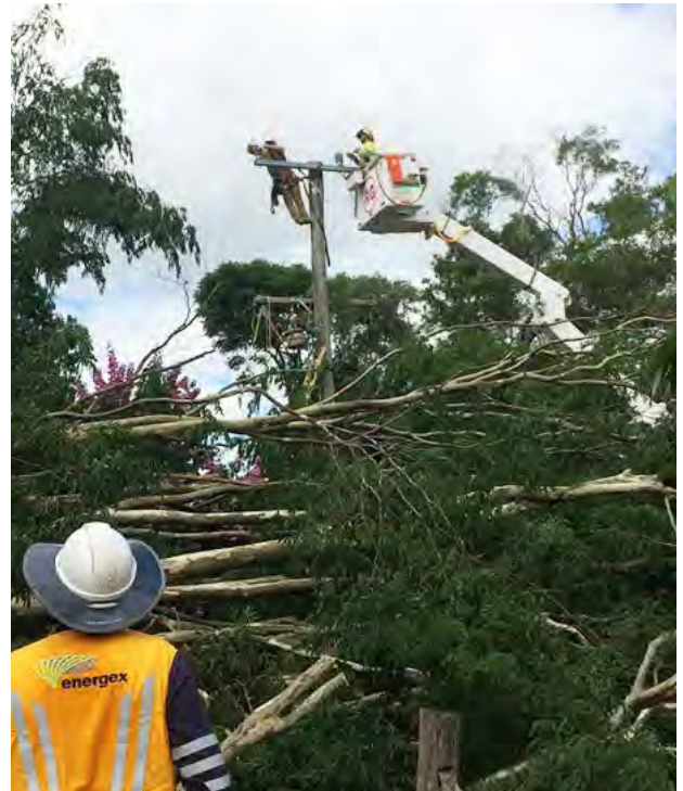
Crews working on powerlines
