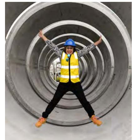
Cr Bradley with some of the giant stormwater pipes being laid in Rochedale South.
