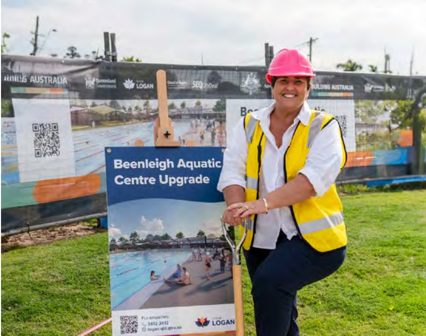
Cr Murphy turns the first sod to launch construction of a new 50-metre pool in Beenleigh.
