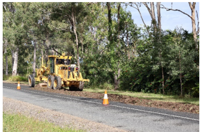
Figure: Typical grader clearing out the shoulder of the road.
