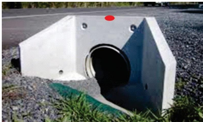
Figure 18 - End Structure Headwall
