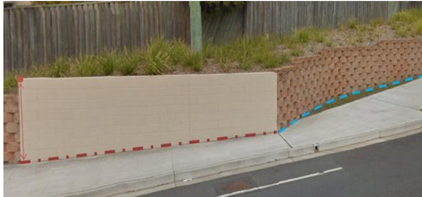
Figure 13 - Example of Retaining Wall
