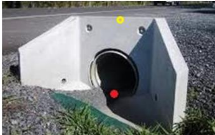
Figure 43 - Example of an outfall headwall
