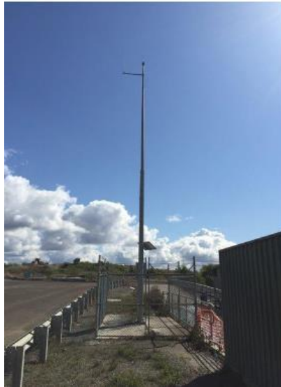
Figure 44 - Example of a Monitoring Station
