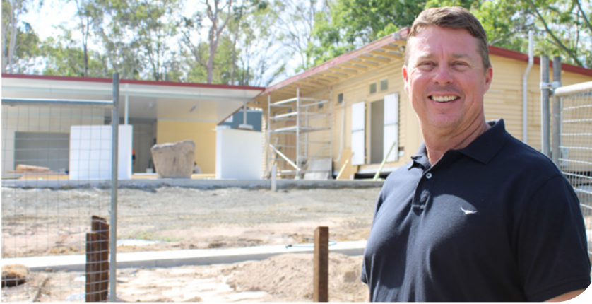
Councillor Scott Bannan inspects the RSL relocation works at Jimboomba Park.
