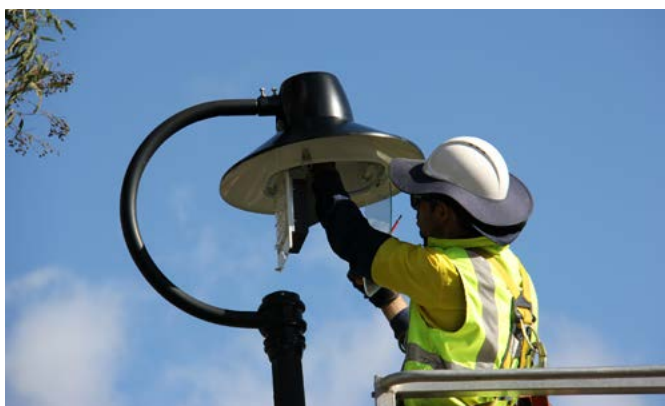
Retrofitting pathway lights with LEDs
