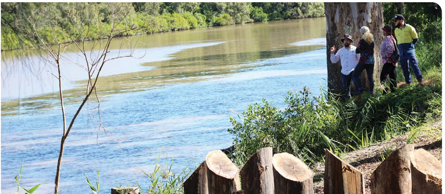
Log pile fields were installed during a community planting day at Logan River Parklands on 12 June 2021.
