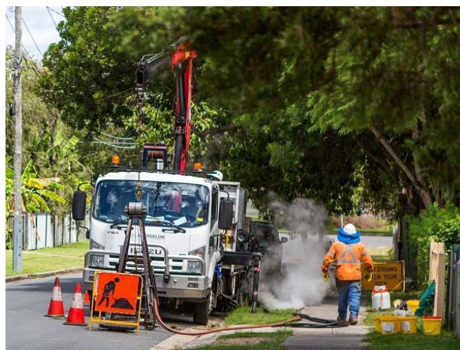
Pipeline relining in progress
